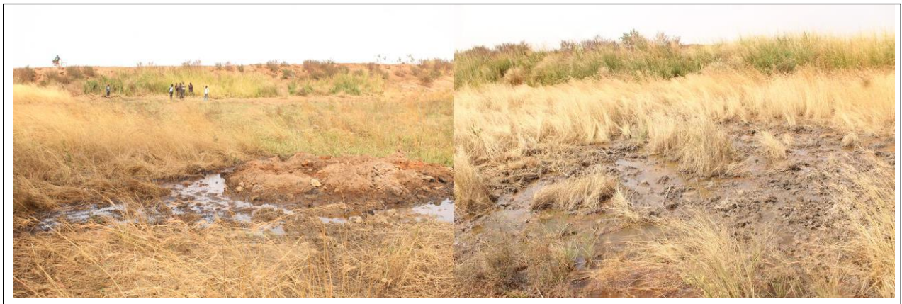
Plate 2. Water oozing out of the ground a distance away from behind the Vunania dam
