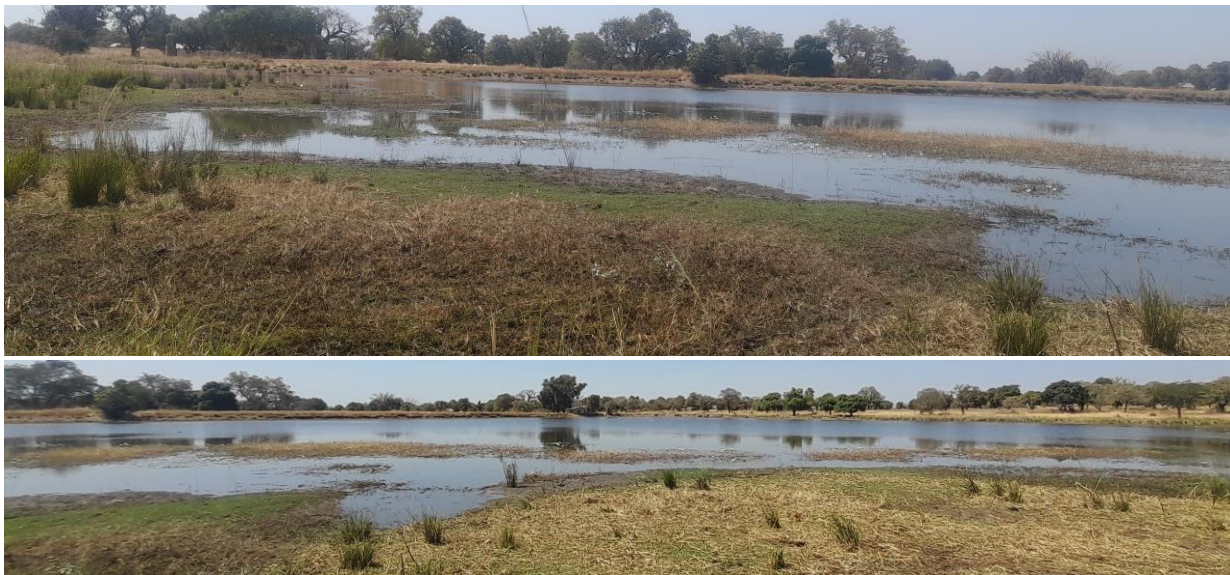
Plate 5. The Brigade reservoir in Vunania constructed using community labour in 1963, still sustainably serving its purpose.
