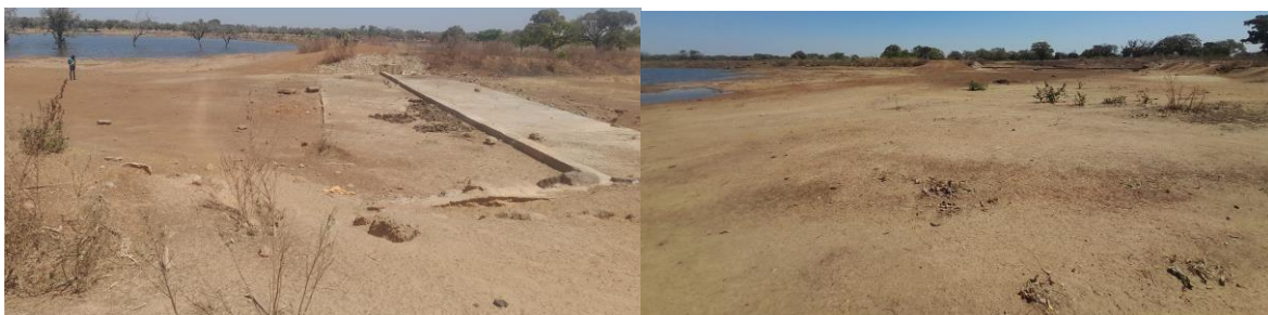
Plate 3. Spillway of the Vunanai dam and the high elevation of the impounded area leading to the spill
