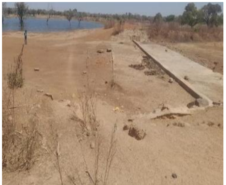
Seemingly high spill way approach.
