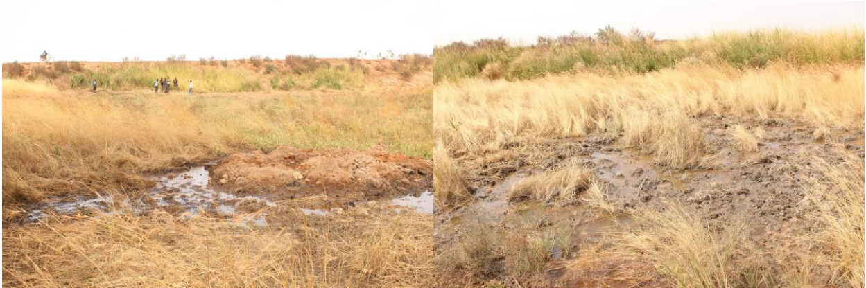
Water oozing out of the ground a distance away from behind the Vunania dam
