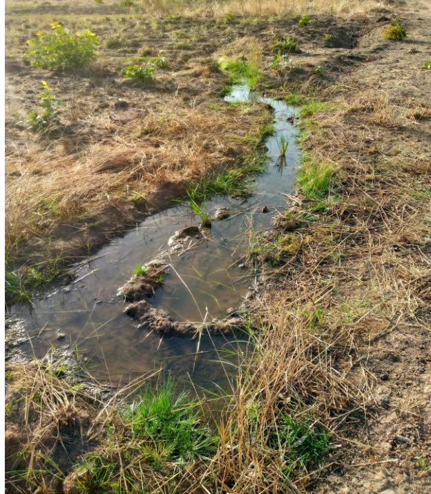
leakages in the irrigable area along the main pipeline
